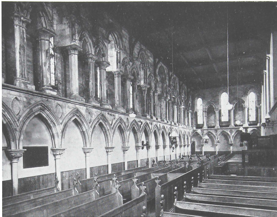
COLDINGHAM PRIORY: INTERIOR LOOKING EASTWARD, BEFORE THE RESTORATION
