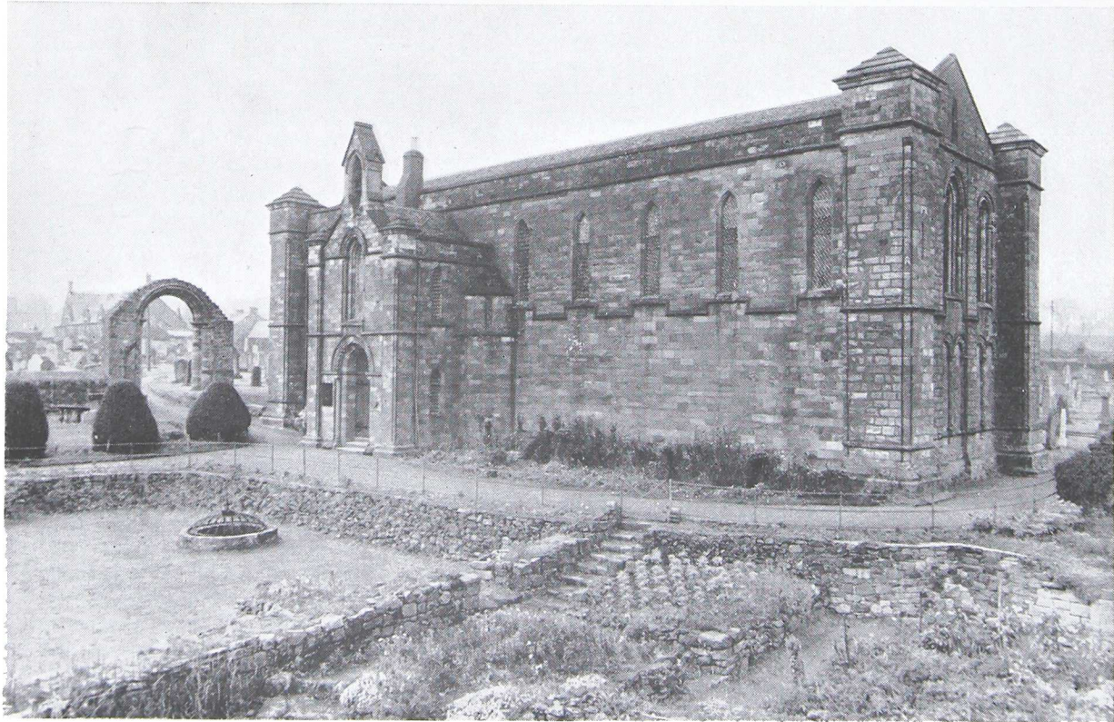
COLDINGHAM PRIORY: FROM SOUTH EAST, SHOWING CLOISTER GARTH, WELL, AND ARCHWAY TO SOUTH AISLE
