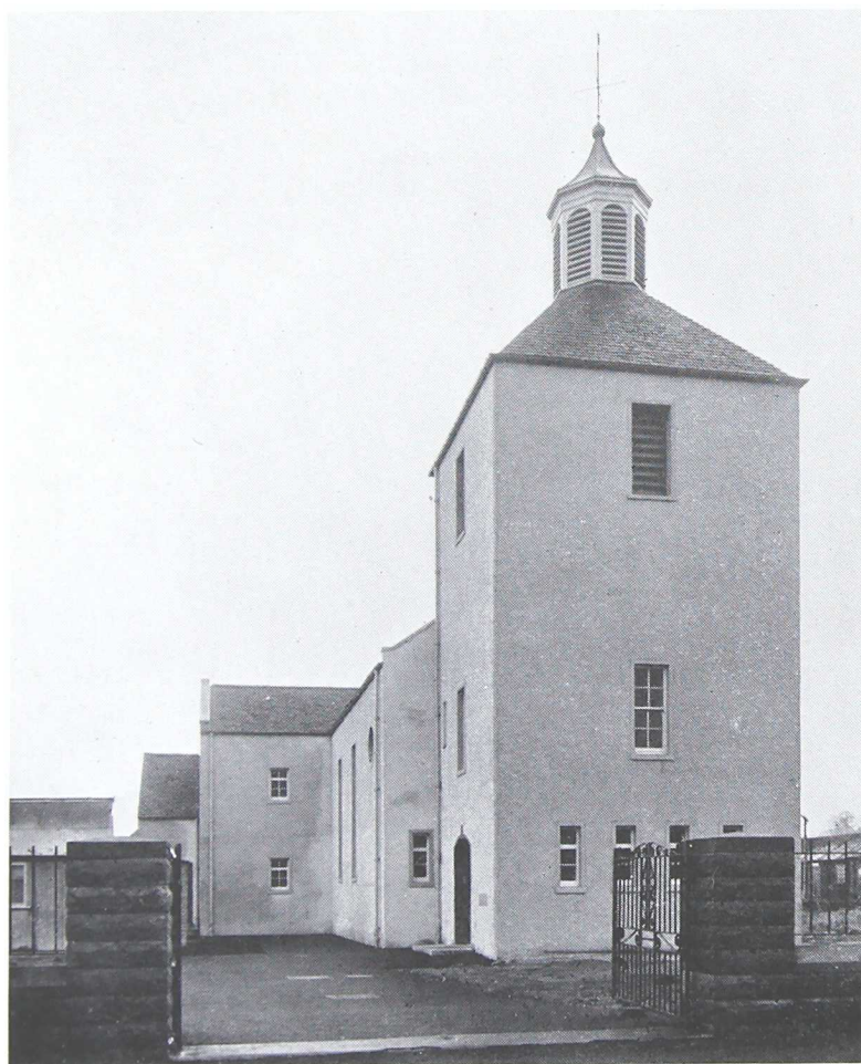
COLINTON MAINS CHURCH : EXTERIOR FROM WEST.
